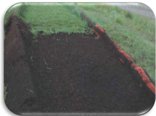
Figure 8 - Compost Blanket Application.
