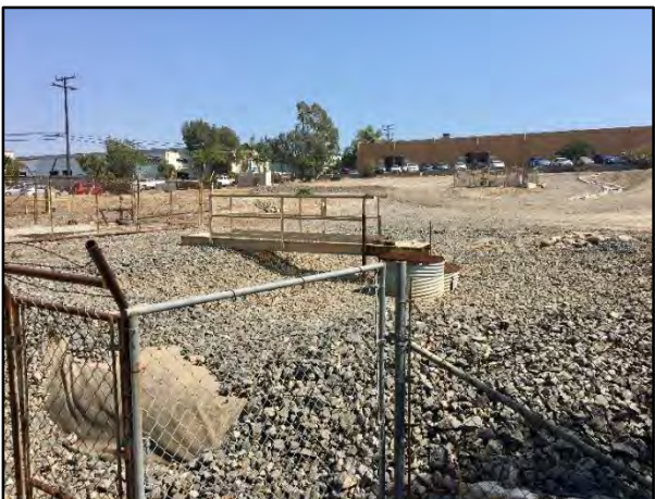
Permanent Sediment Control Device
