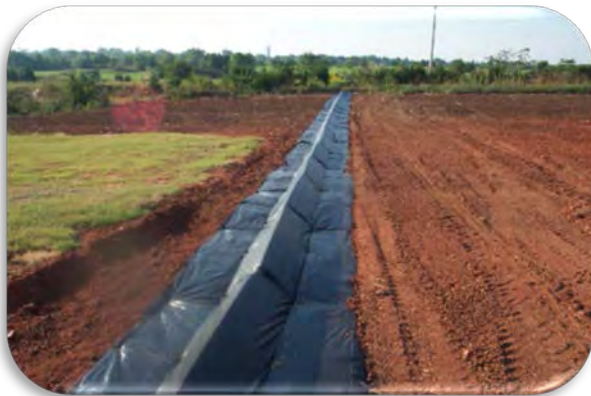
Figure 7 - Silt Dike Application.
