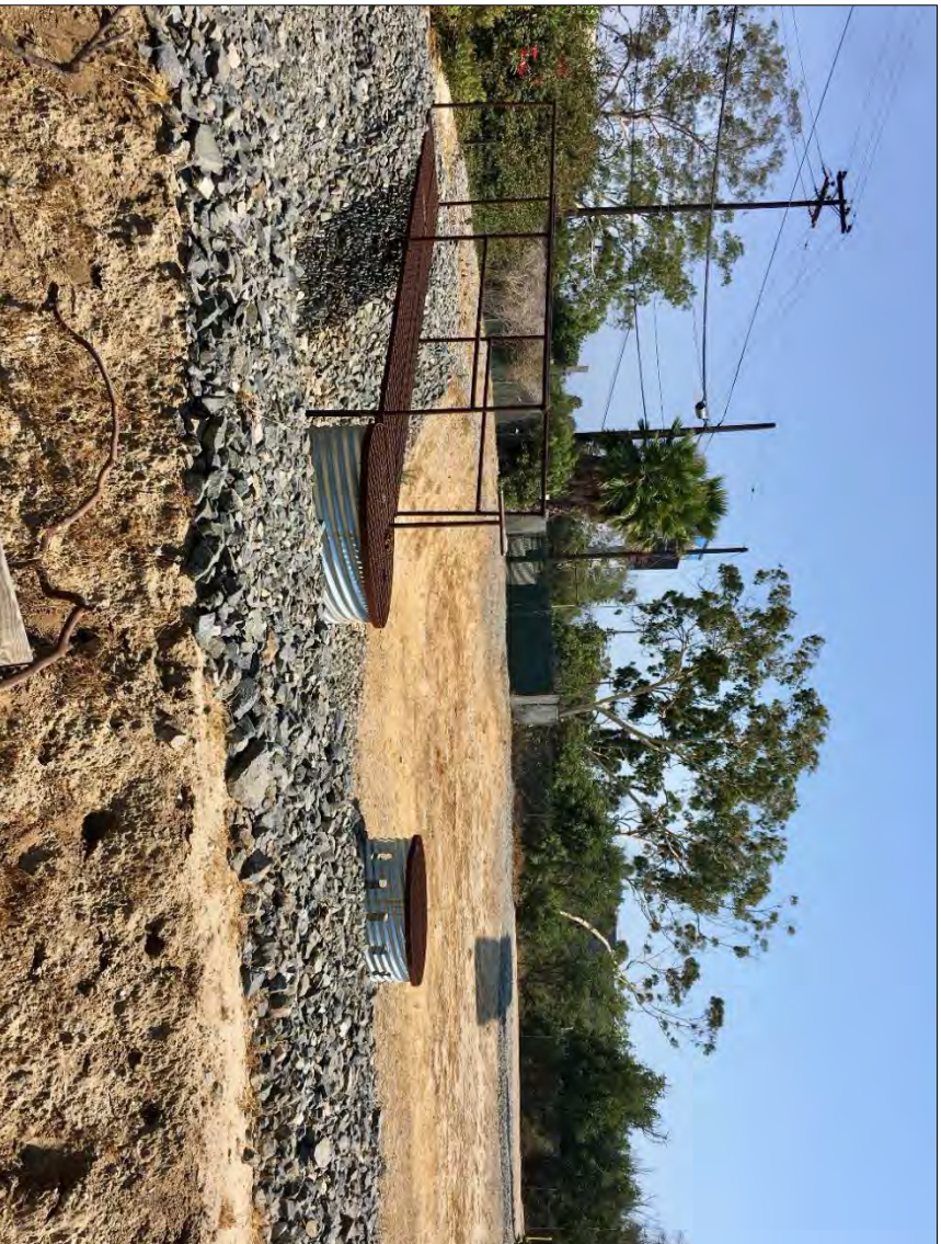
Sediment Control Device (Vacant parcel adjacent to Target)
